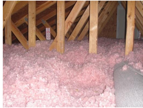
Figure 14 Attic insulation adequate
