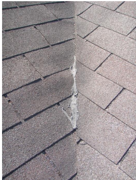
Figure 17 Calking on valleys
