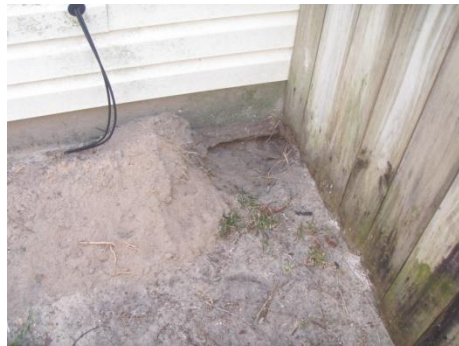
Figure 11 Back fill needed.
